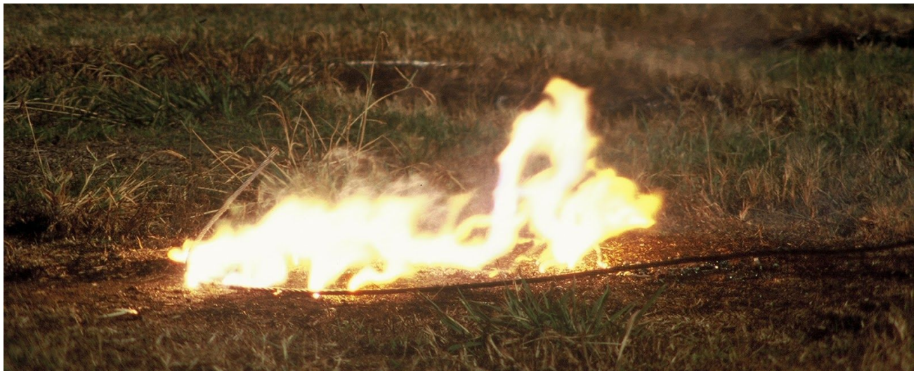
A live, downed conductor starting a fire
